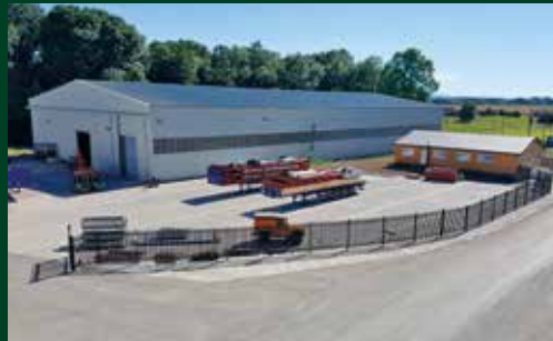
Shobdon Steel Fabrication Site
